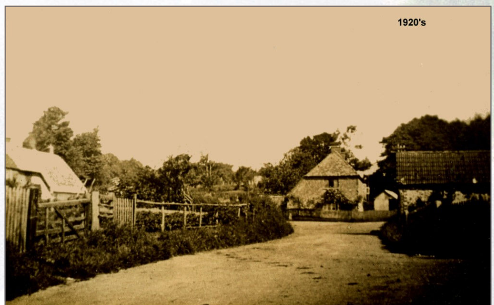
"Hope Cottage" - Livery Road, West Winterslow
